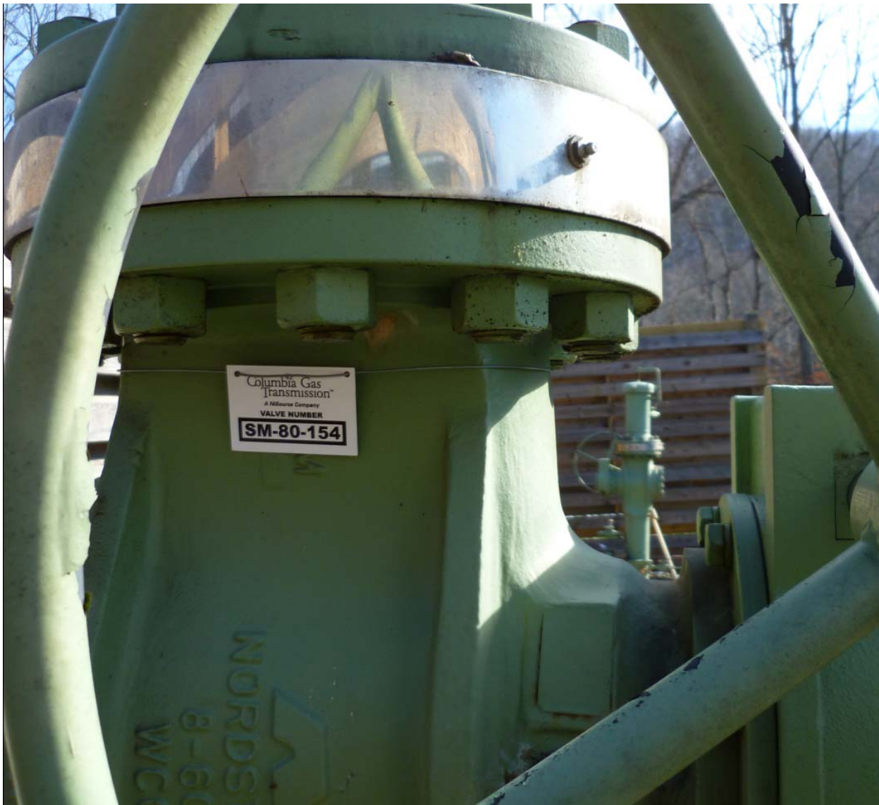
Photos of SM-80 – Martha's Valve Setting – Installed Valve Tags
