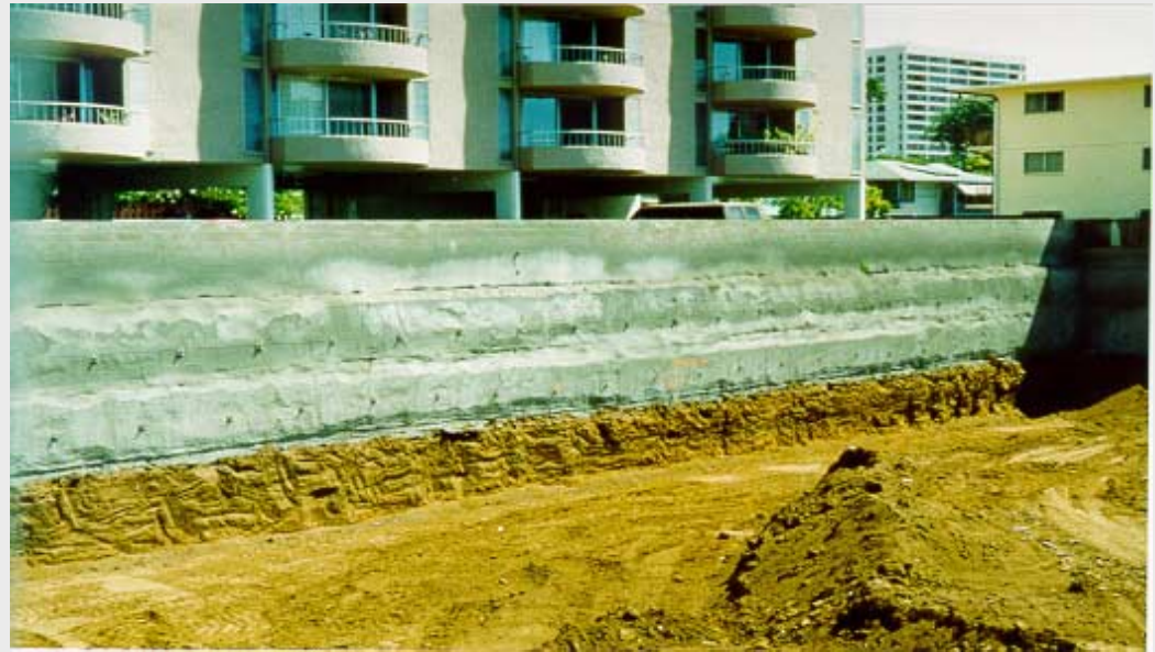
Example of the use of Soil Nailing in stabilization of cuts.
