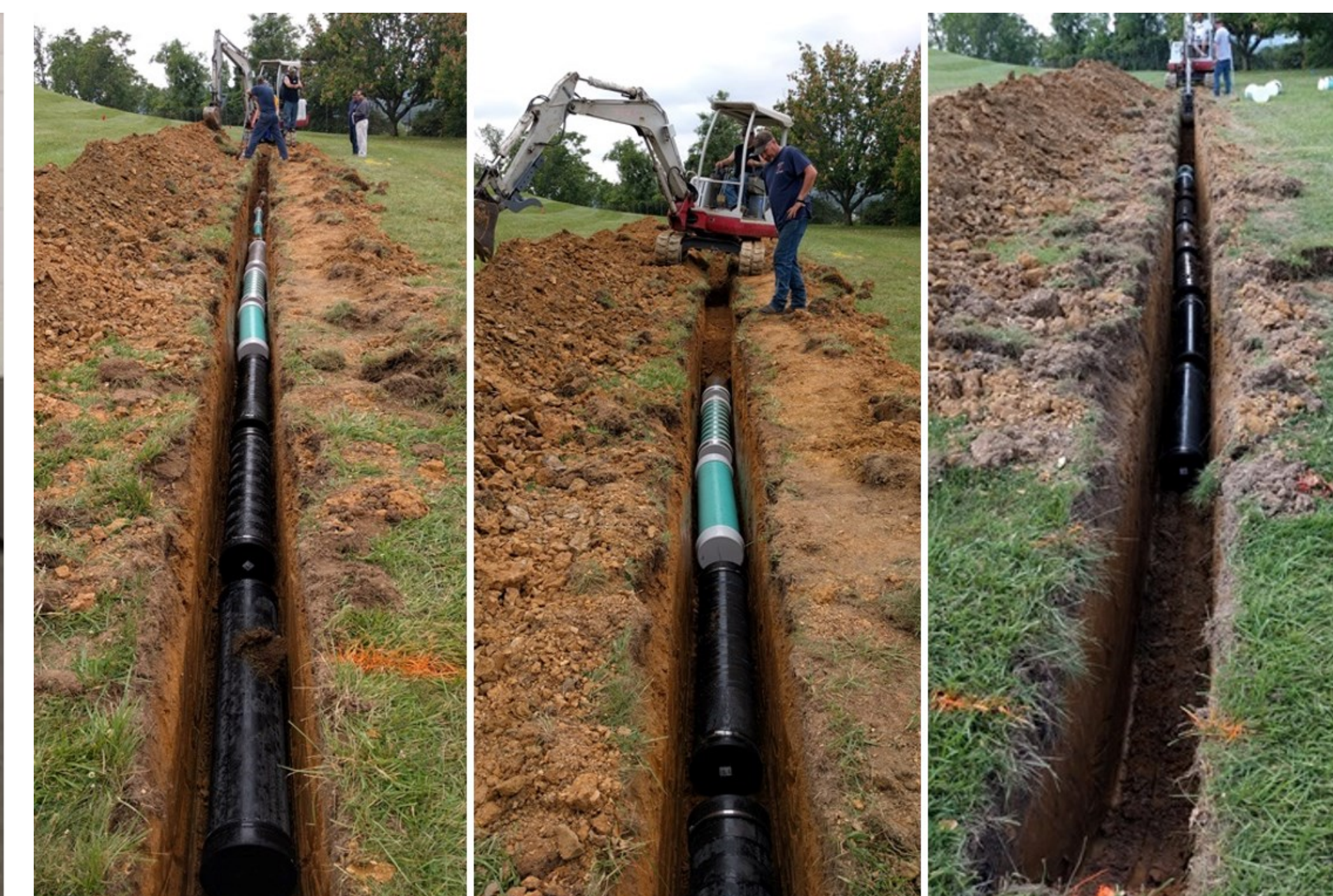
Figure 4. Pipe samples being buried.
