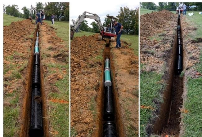
Figure 4. Pipe samples being buried.
