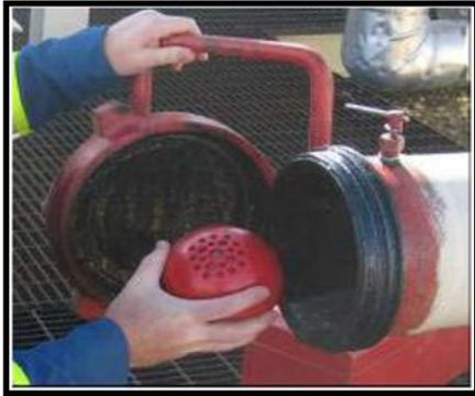
Internal Liq/N-Gas LDS transferred from the water pipeline industry
