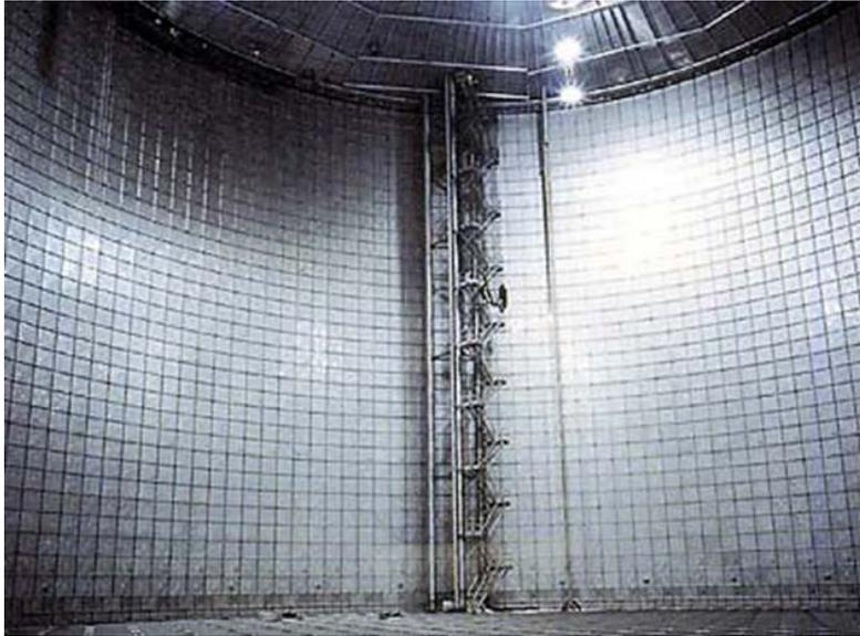
**Membrane Tank** - A tank that uses a thin metallic liner as the inner tank. Unlike a conventional metal tank (which is self-supporting), a membrane cannot support its own weight and must be supported by other means.
