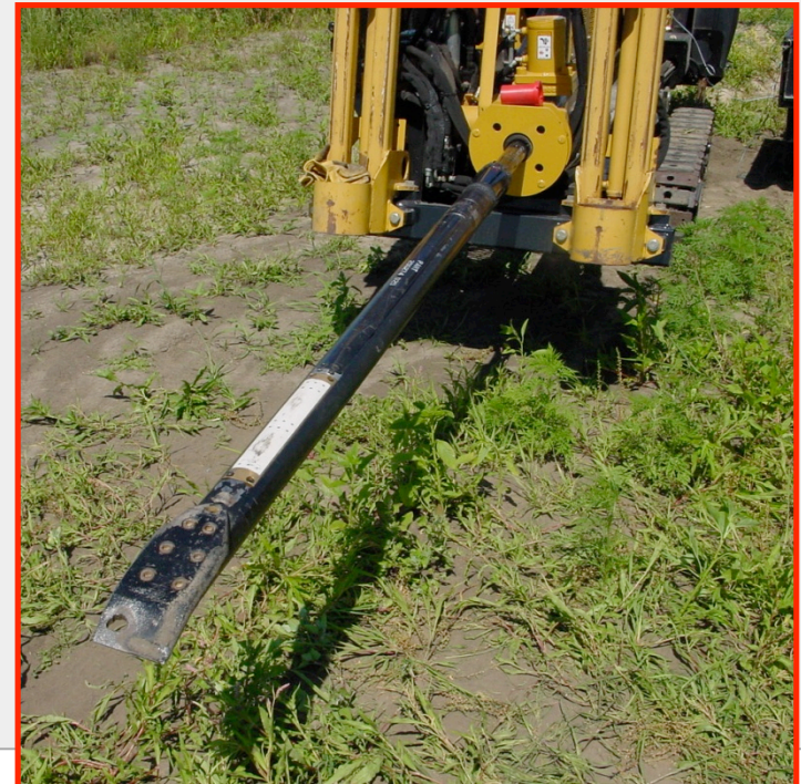
Radar mounted on 18x22 drill
