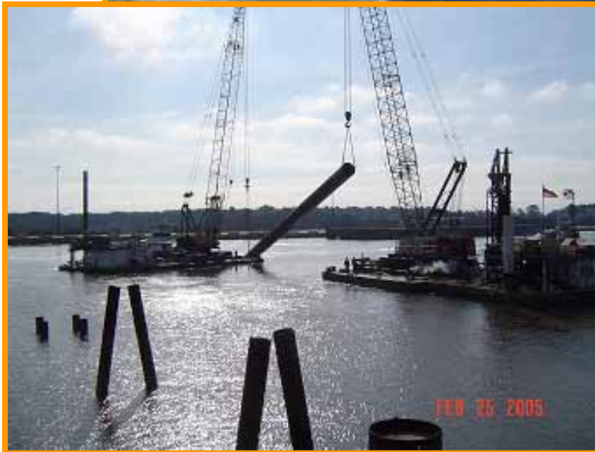
Dock Monopile Installation
