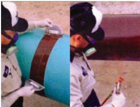
Figure 5.5 – Powercrete® pipeline coating application ( http://www.petropages.com/vendors/v19548.htm )
