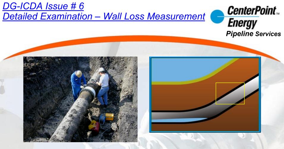
Research shows water may likely accumulate between inclination onset and 1/3<sup>rd</sup> up slope – angle in pipe may possibly affect signal strength – when using GUL, there is a dead zone – what method of wall loss thickness measurement is ideal (handheld UT grid? - over what length and circumference)?
