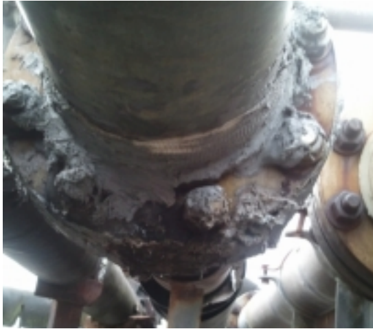
Figure 2: Photograph of a flange that has been leaking long enough to cause extensive corrosion.
