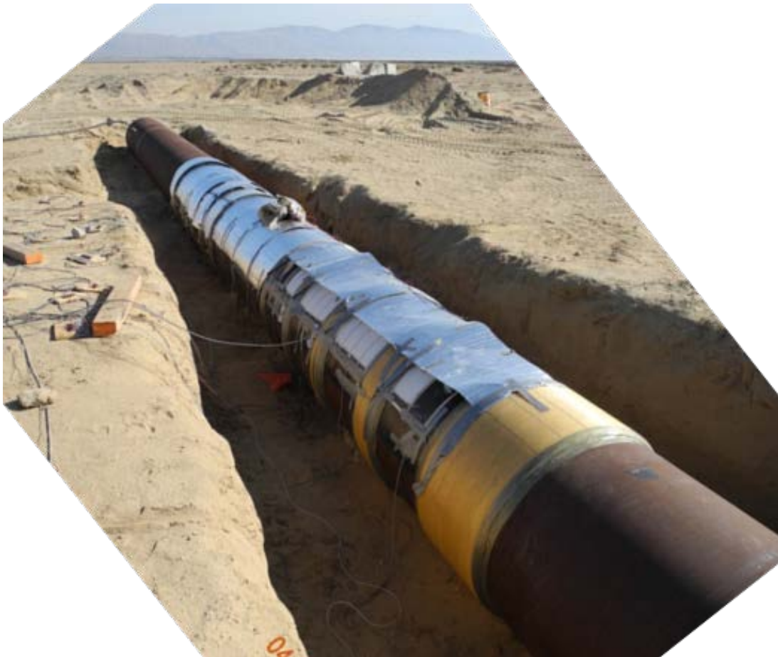
Figure 15 Test pipe prior to test start
