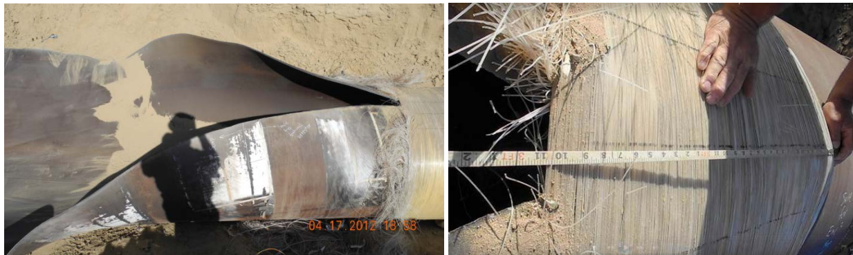
Figure 17 Crack Arrest at 5th Arrestor on Pipe #693
