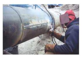
Despite advances in mechanized welding technology, manual welding using cellulosic coated electrodes is widely utilized throughout the world
