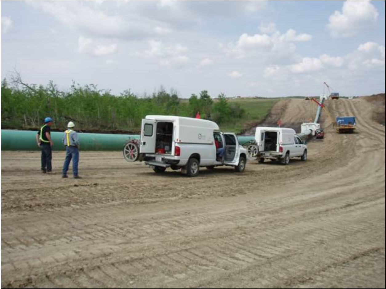
Figure 12. EWI Truck Following UTQ Truck Performing AUT Scans for TCPL
