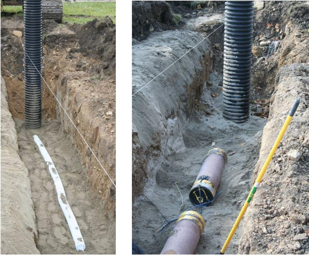
**Figure 63. Drainage pipe installed prior to laying of the 8 inch pipeline sections in sand backfill (left); pipeline sections in partially filled trench (right). Upright corrugated stack houses a sump pump to remove drained water.**
