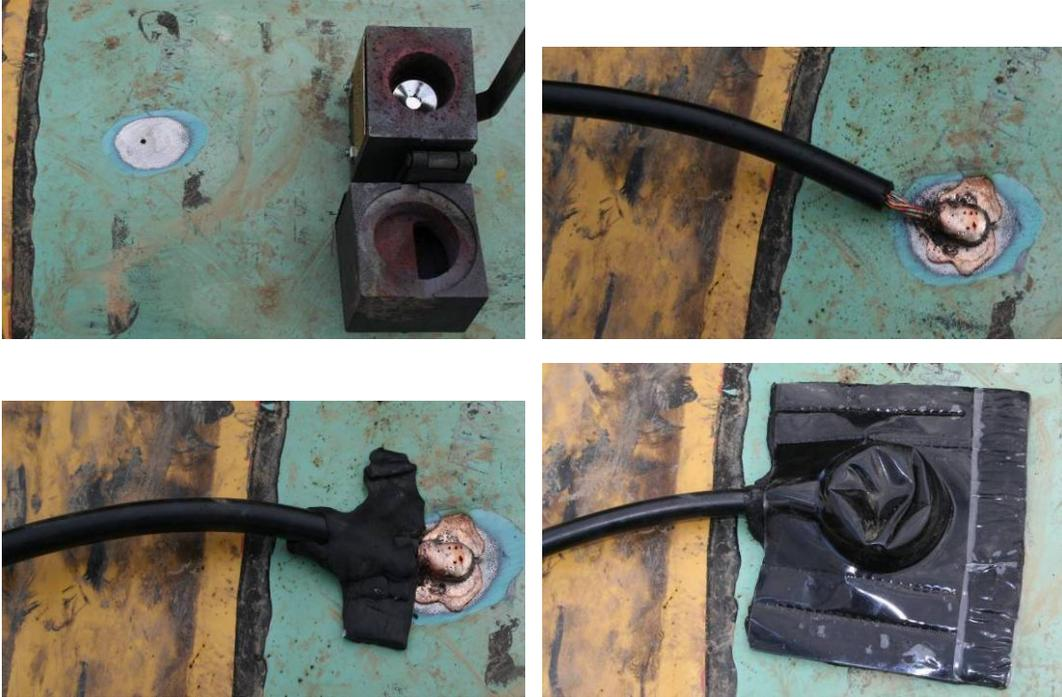
**Figure 60. Installation of cable leads.**
