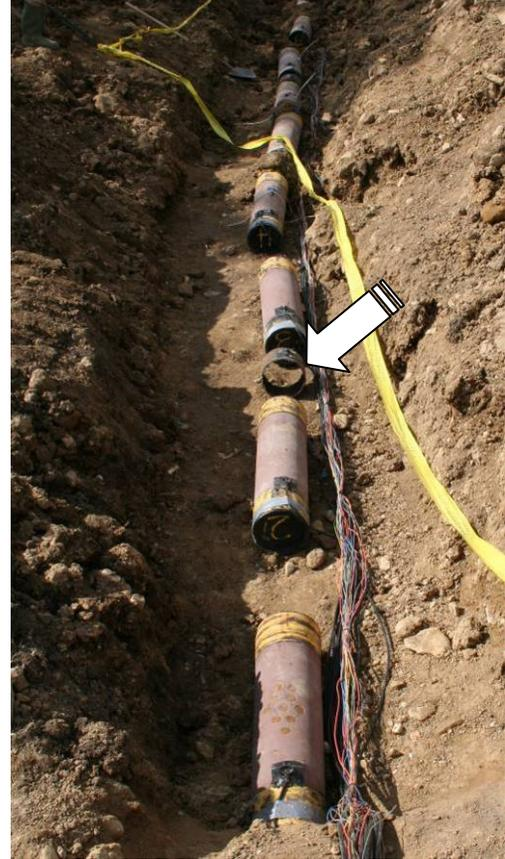
**Figure 61.** Installation of first 9 sections (20 inch line on the left, 8 inch line on the right). Note bare pipeline sections indicated by arrows.
