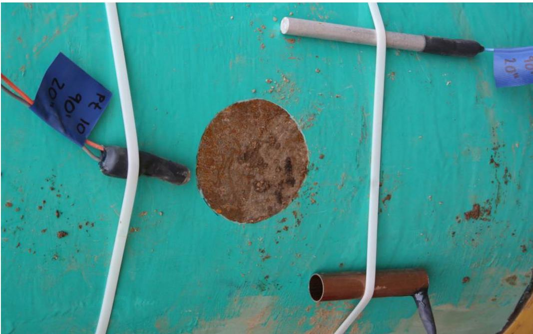
**Figure 58. Reference electrode (left), magnesium electrode (upper right) and copper electrode (bottom right) strapped to the 20 inch pipeline section prior to installation.**
