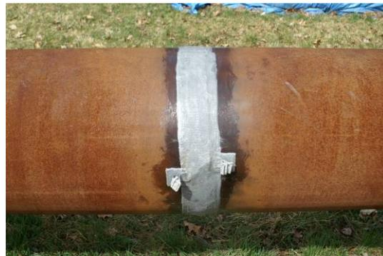
Figure 4. Wax coating applied over MsS assembly
