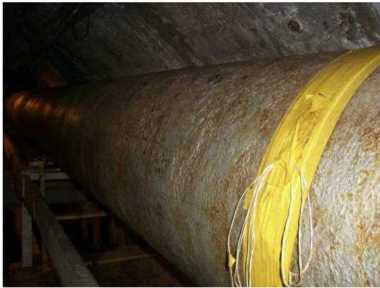
MsS installed on 26" gas pipeline in the Astoria Tunnel
