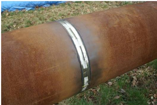
Figure 1. Alloy strips bonded to pipe with epoxy
