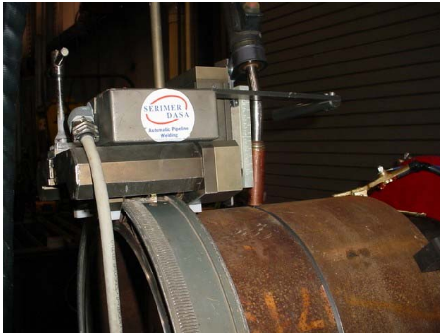
Figure 6. Serimer Dasa STX Pipeline Welding Tractor and Track on 16-in.-Diameter Carbon Steel Pipe
