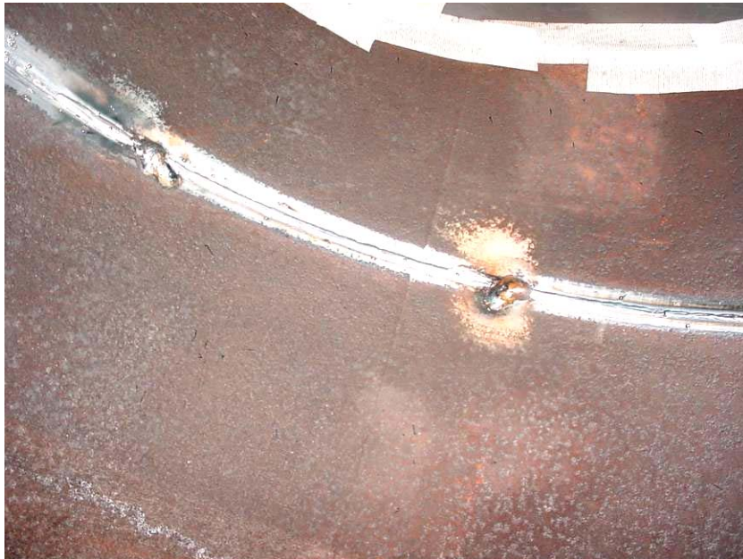
Figure 25. Spin Arc GMAW Weld W13 Showing Root Pass Penetration – 130-180 Degree Downhill
