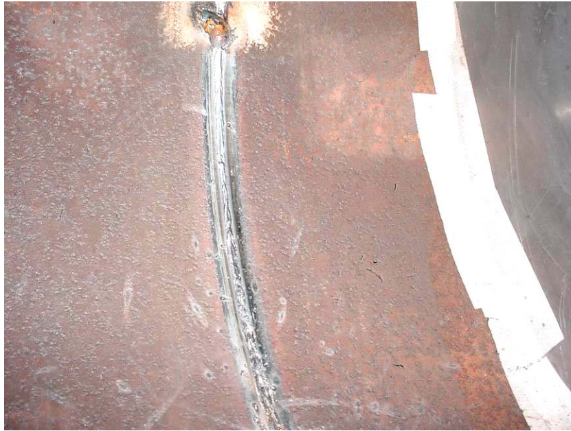
Figure 24. Spin Arc GMAW Weld W13 Showing Root Pass Penetration – 90-160 Degree Downhill
