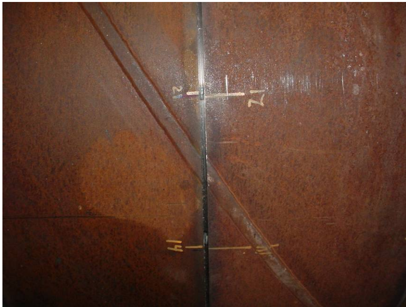
Figure 49. 36-in.-Diameter X80 Pipe Joint Showing Crossing Seam for Spiral Wound Pipe Welded with SAW
