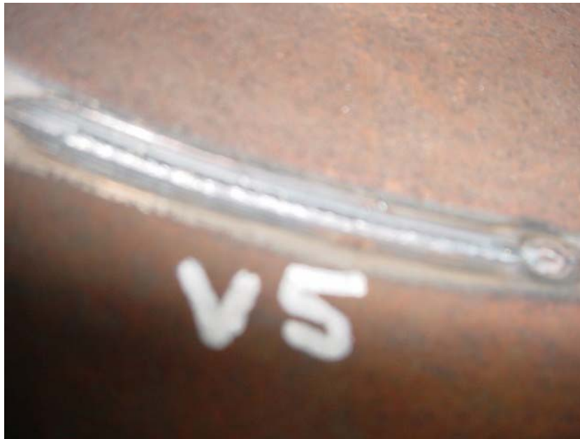
Figure 16. GMAW-VP Weld V5 – Penetration Bead on Inside of Pipe
