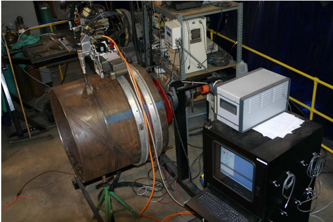
Figure 13. GMAW-RE Torch Setup at 12:00 o'clock Position on 36-in.-Diameter X80 Pipe, Also Showing Industrial Controller
