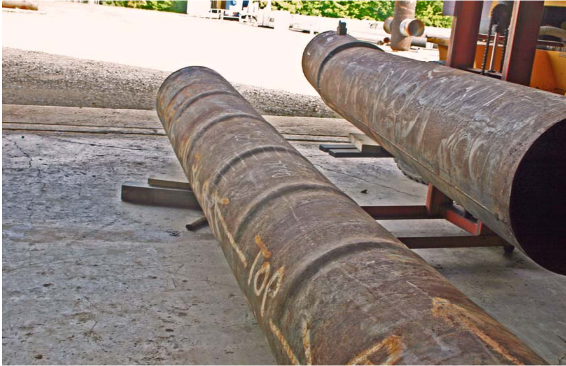
a) views of segments A (left) and B (right)
