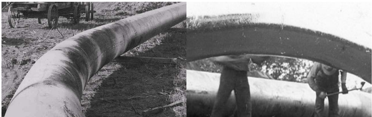
Figure A6. Typical bend produced by the hot wrinkle bending apparatus in Figure 5 – very little pipe distortion is evident
