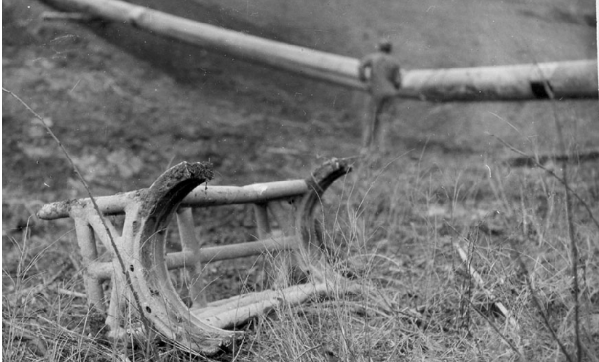
Figure A3. Fabricated frame used as fulcrum in making cold wrinkle-bends (circa 1930s) – view in background shows a wrinkle so produced being inspected
