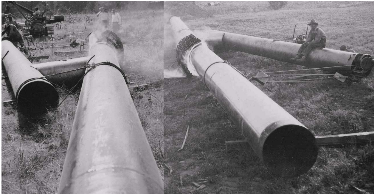
a) setup with fulcrum and tie-line b) during heating, winch in foreground Figure A4. Views of one hot wrinkle-bending fixture (circa 1931)
