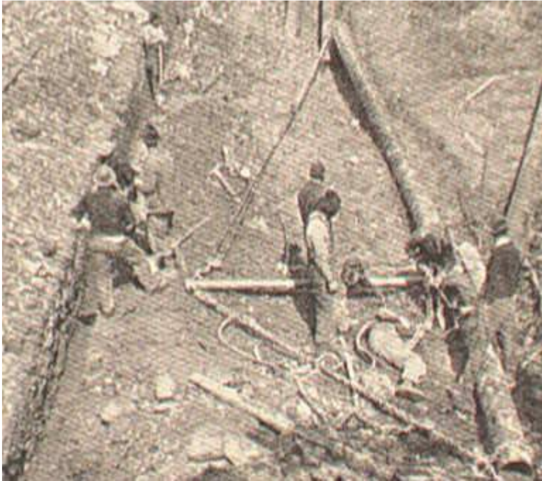
Figure A7. A-Frame wrinkle bending fixture (circa 1930s).
