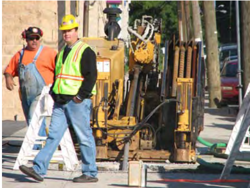
Horizontal Drilling Machine Dec. 06 – Bronx, NY
