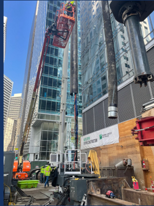
DFOS monitoring of the deep foundation of a high rise building in San Francisco
