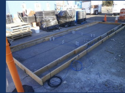
DFOS installation for concrete pavement (with UC Davis)
