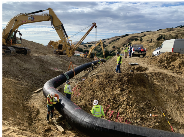
Figure 27: Outer wrap application
