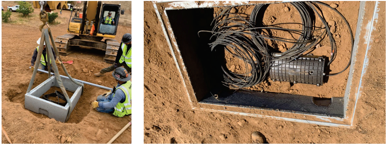
Figure 28: Pull box installation
