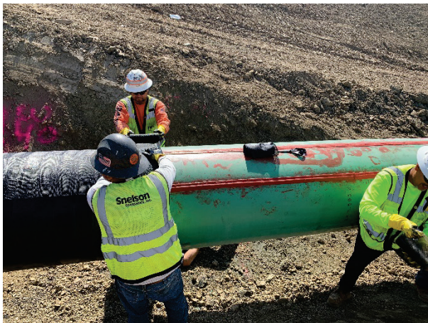
Figure 27: Outer wrap application
