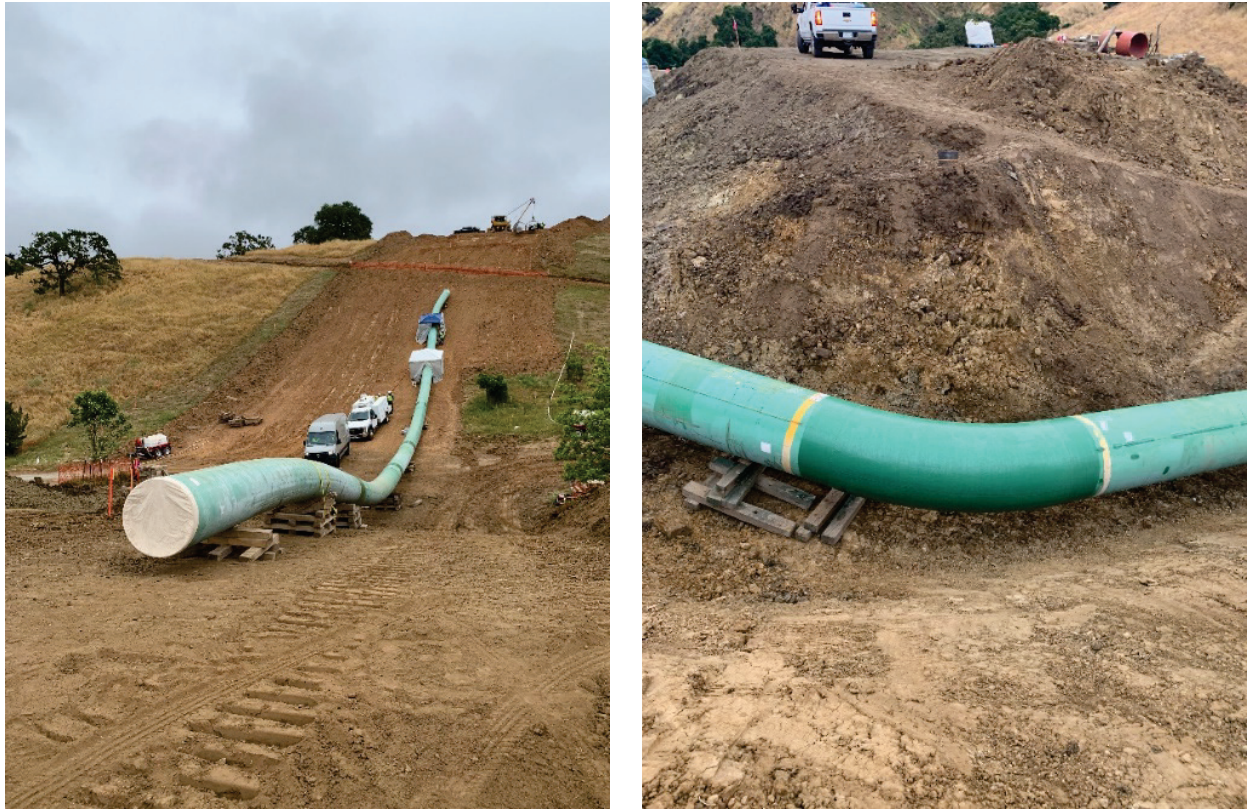
Figure 23: Photos of (a) 220-foot-long straight segment; (b) 60-foot-long elbow segment
