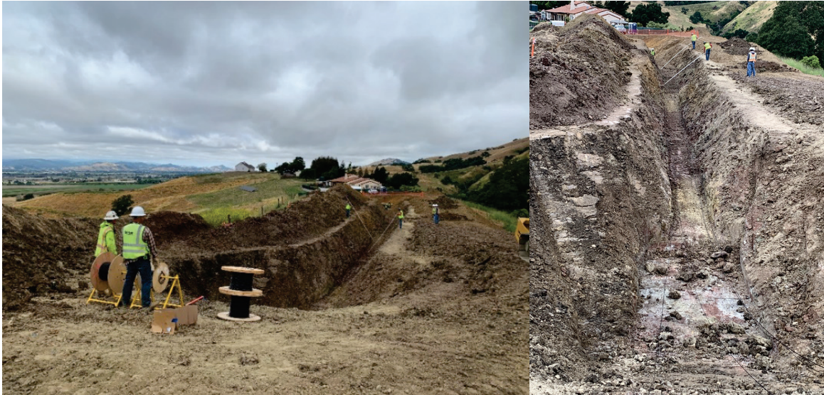
Figure 22: Fiber optic sensor installation in the trench
