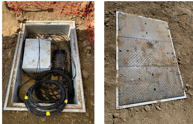
Figure 30: Pull box after all work is completed
