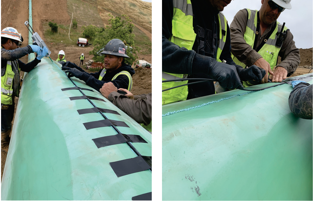
Figure 24: Adhesive material application
