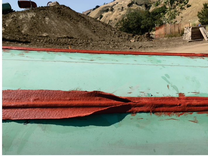
Figure 26: Wax tape application
