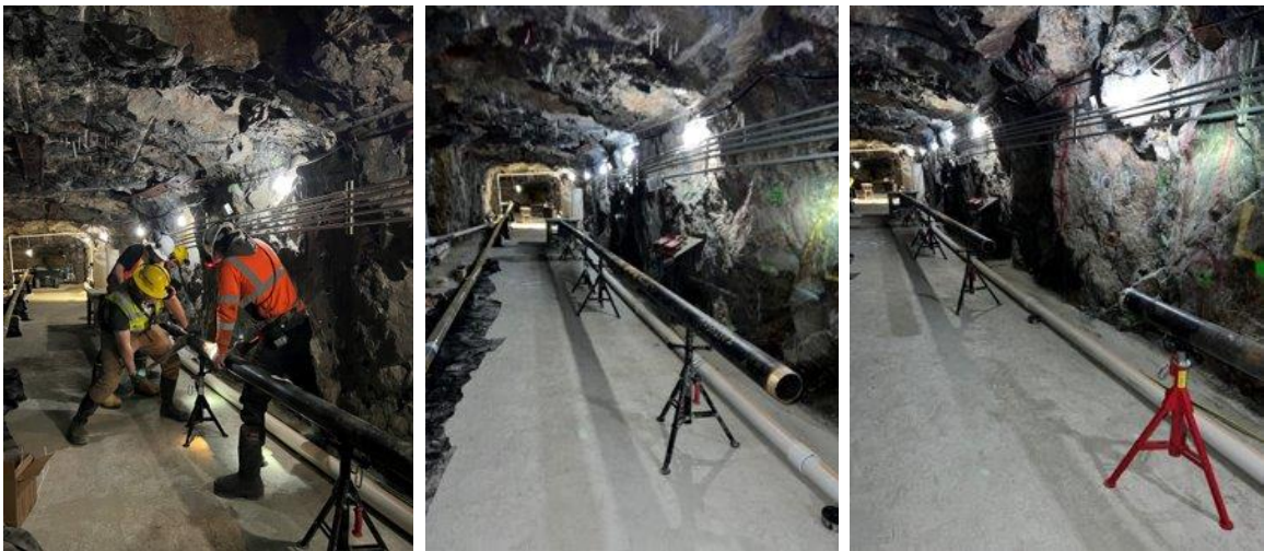
Fig. 4. Photograph of the steel pipeline during and after the construction. A 1 m gap is left for testing different defects in Tasks3-6.
