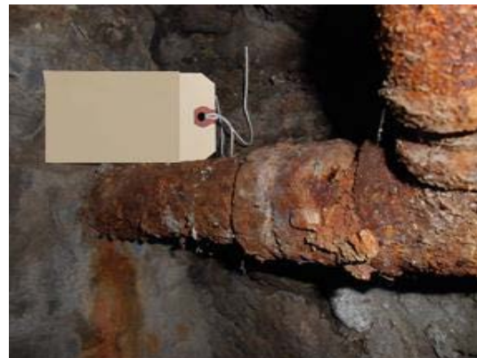
(b) General rust build-up with pitting near fitting
