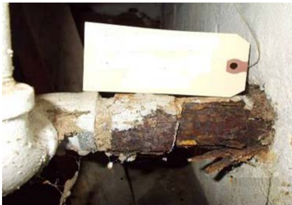
(a) Flaking of pipe surface indicating metal wall loss
