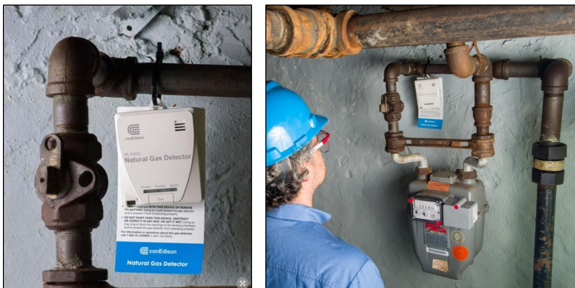
Figure 13. ConEdison new Cosmos ML-310 natural gas detector
