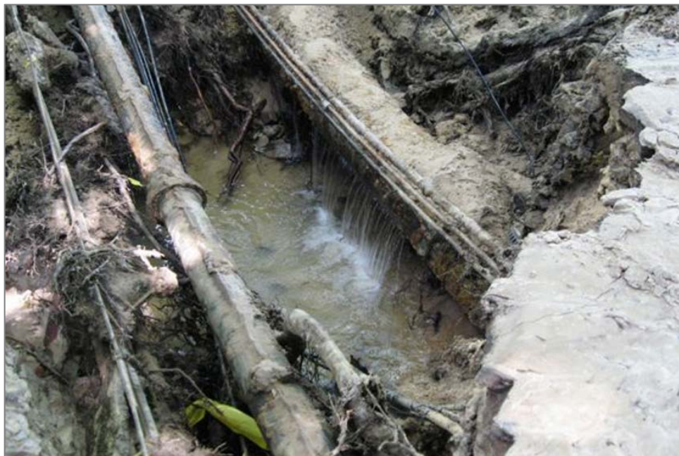
Figure 5. Cast iron cast iron gas pipe in a congested joint trench.
