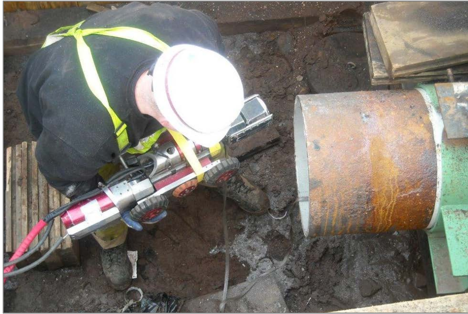
Figure 4. Large diameter cast iron gas pipe about to undergo video inspection.
