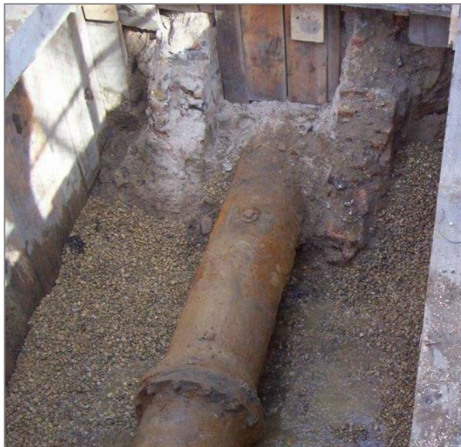
Figure 3. Cast iron gas pipe installation showing flange and bolted connection.
