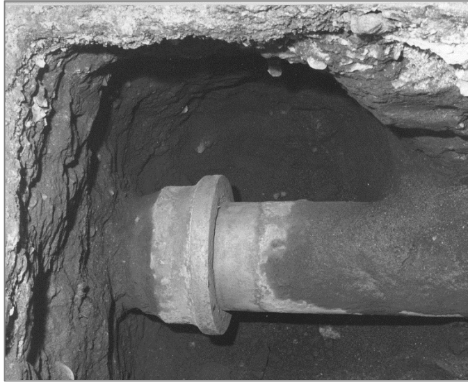
Figure 2. Cast iron gas pipe installation showing bell and spigot joint.
