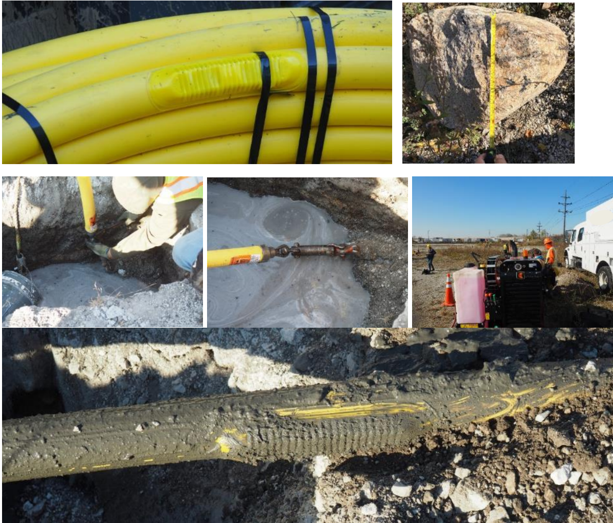
Figure 26: Trenchless installation using HDD equipment at Utility G's training center
