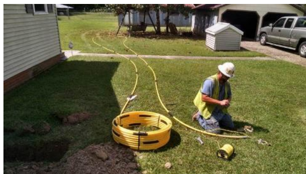
Figure 24: Utility E crews installing ILPP pipe using both trenchless and open trench methods
