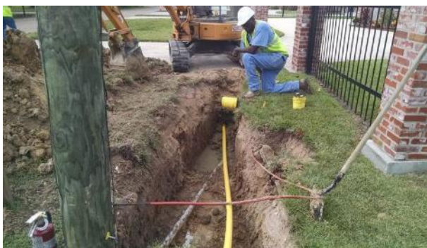
Figure 24: Utility E crews installing ILPP pipe using both trenchless and open trench methods
