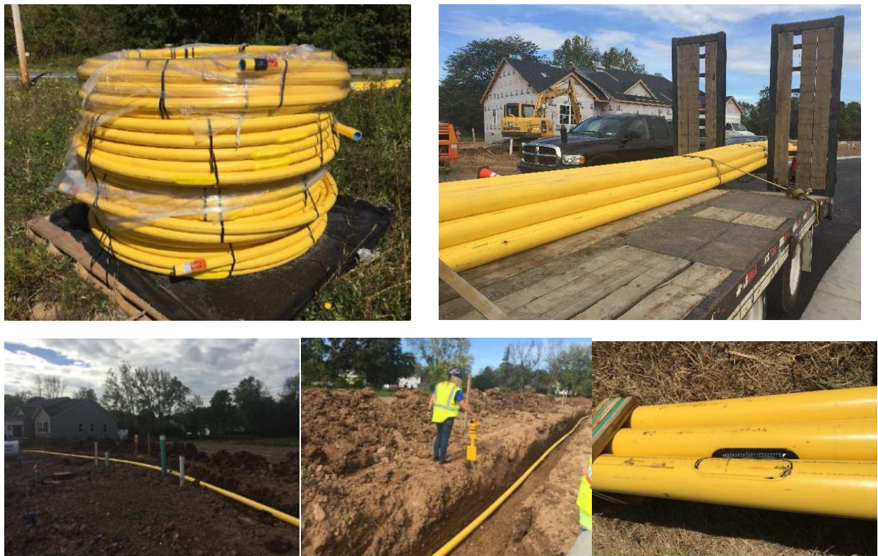
Figure 27: 2" and 4" ILPP installation in Location A
