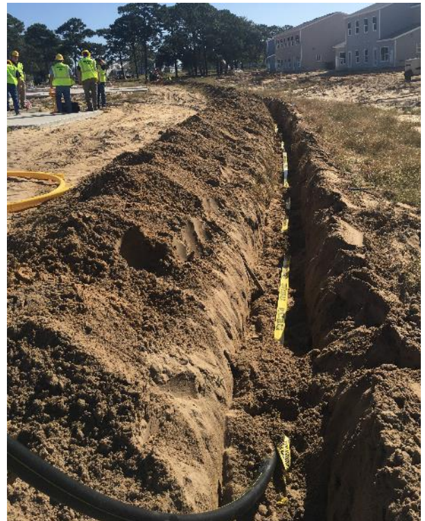
Figure 25: Crews validating the locatability of the installed ILPP at Location A
