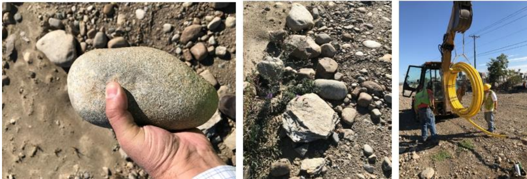
Figure 19: Directional drilling installation of the ILPP in very rocky soils
