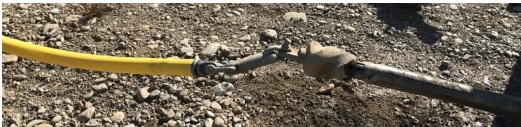
Figure 20: ILPP pipe attached to the back reamer to be pulled into the ground
