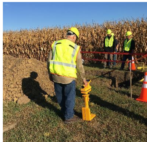
Figure 23: 1" and 2" ILPP trenchless installation at Utility C's training center
