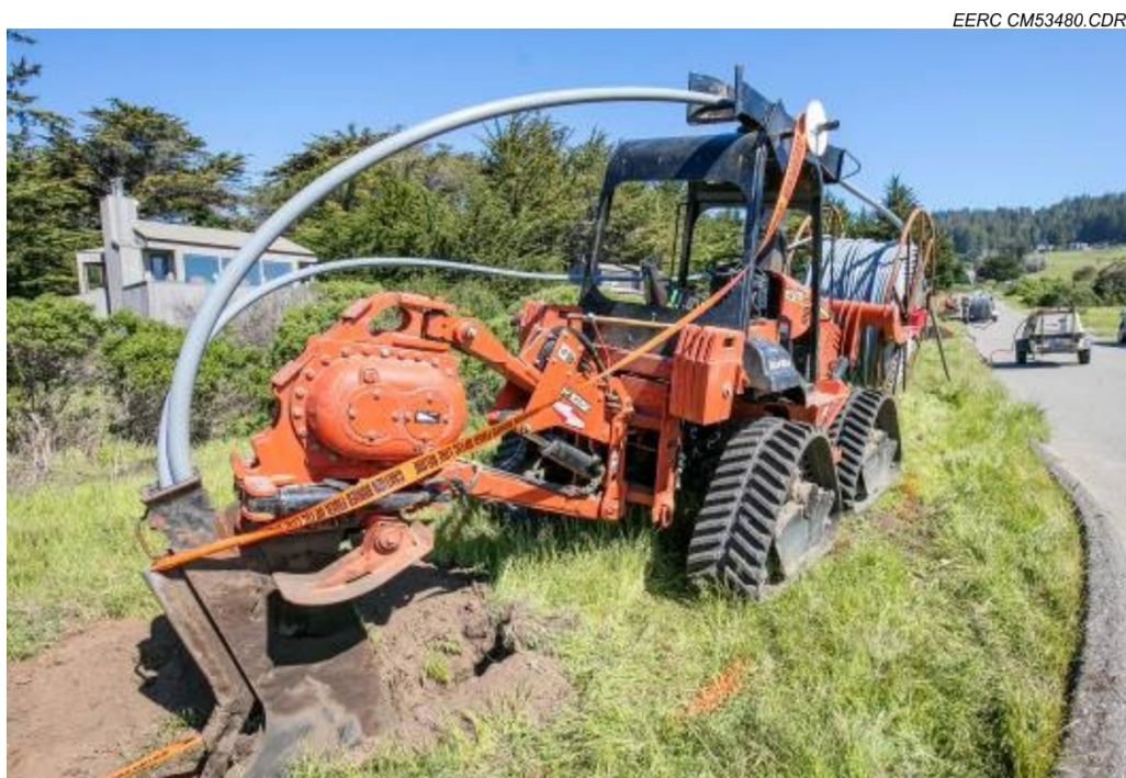
Figure 26. Combined pipe and caution tape trenchless installation (courtesy Sea Ranch Connect).
