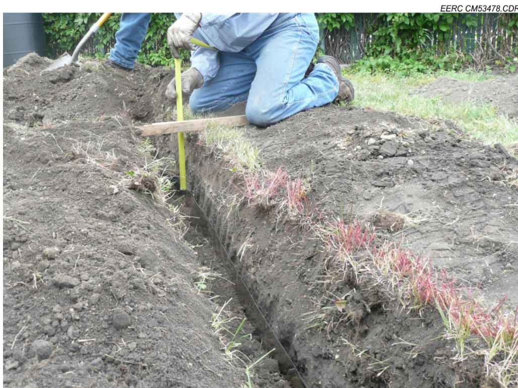
Figure 23. Installation of solid, 5.7-inch laminated tape prototype.
