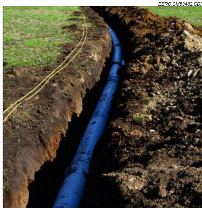
Figure 13. A trenched PVC pipeline [16].
