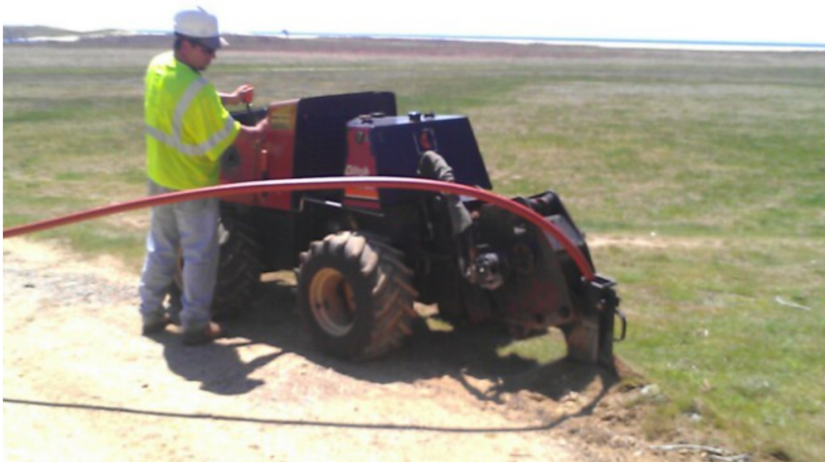
Figure 14. Vibratory plow pipeline installation [17].
