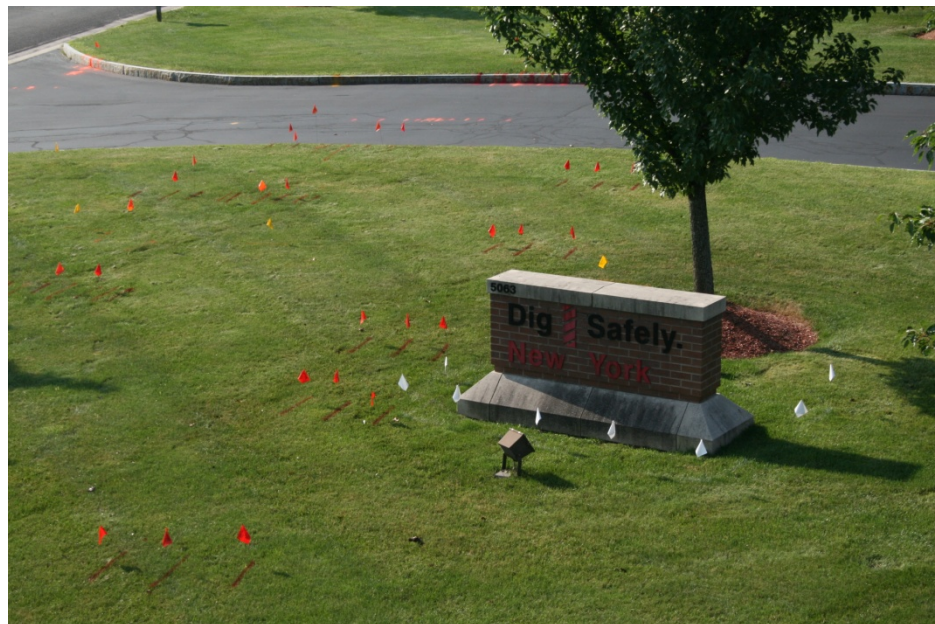
#4 – Marking the Intersection of the Utilities & the Dig
