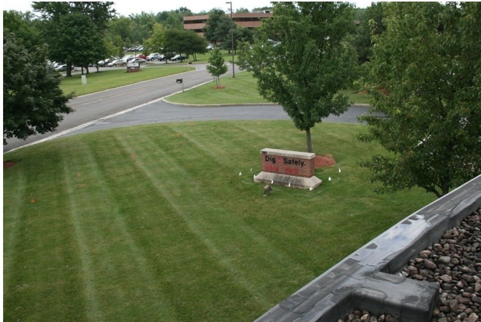
#3 – Verifying the Marking of All Utilities
