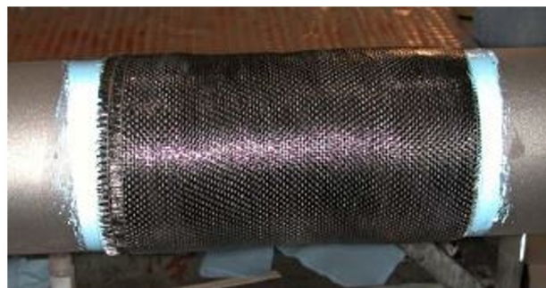
Figure 2.4: Wrapping of wetted out fabric (left) and final repair (right)
