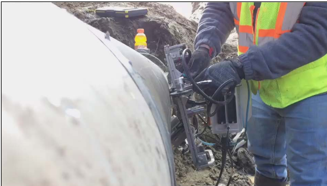
Figure 122. Scanning the pipe
