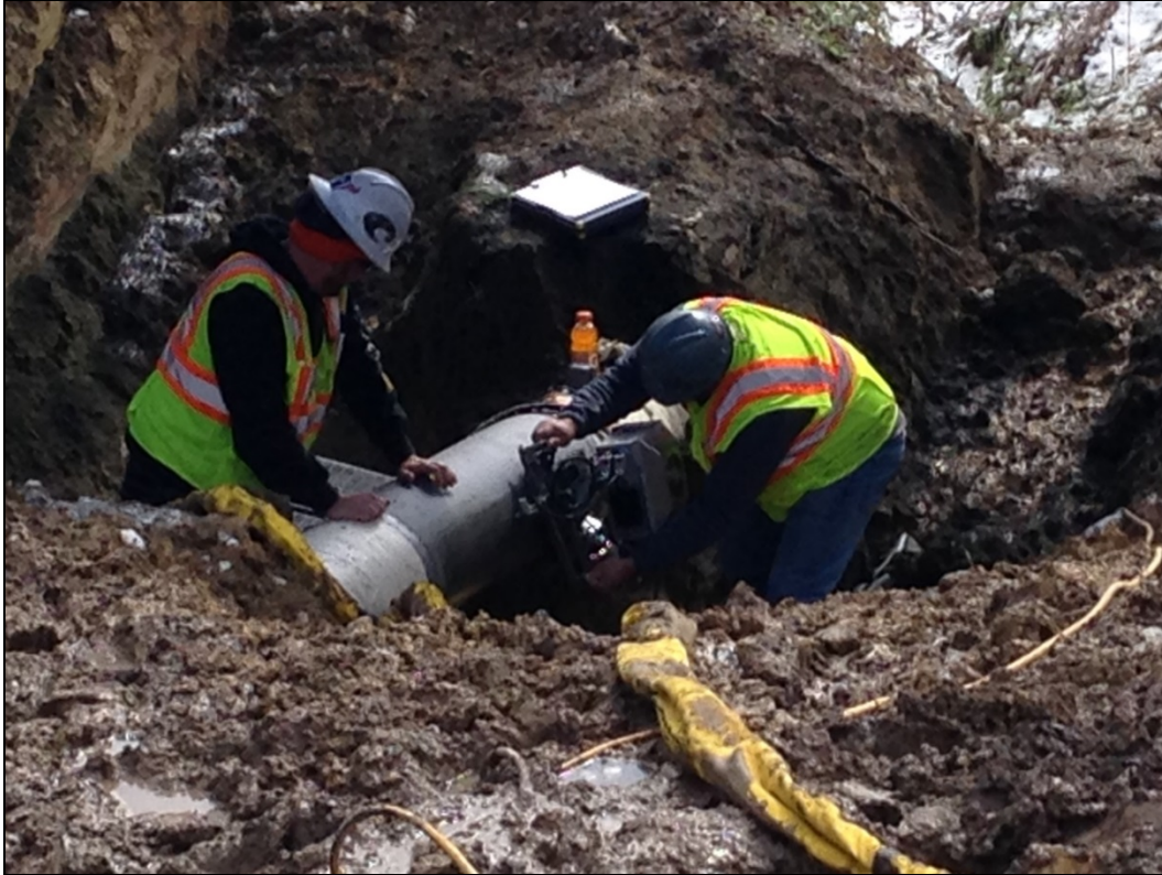
Figure 121. Scanner set up
