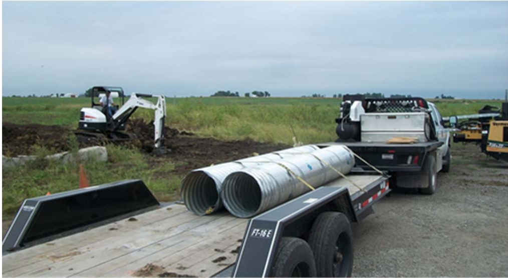
Figure 24 Photograph of 18" culverts to be used as test targets prior to their burial.
