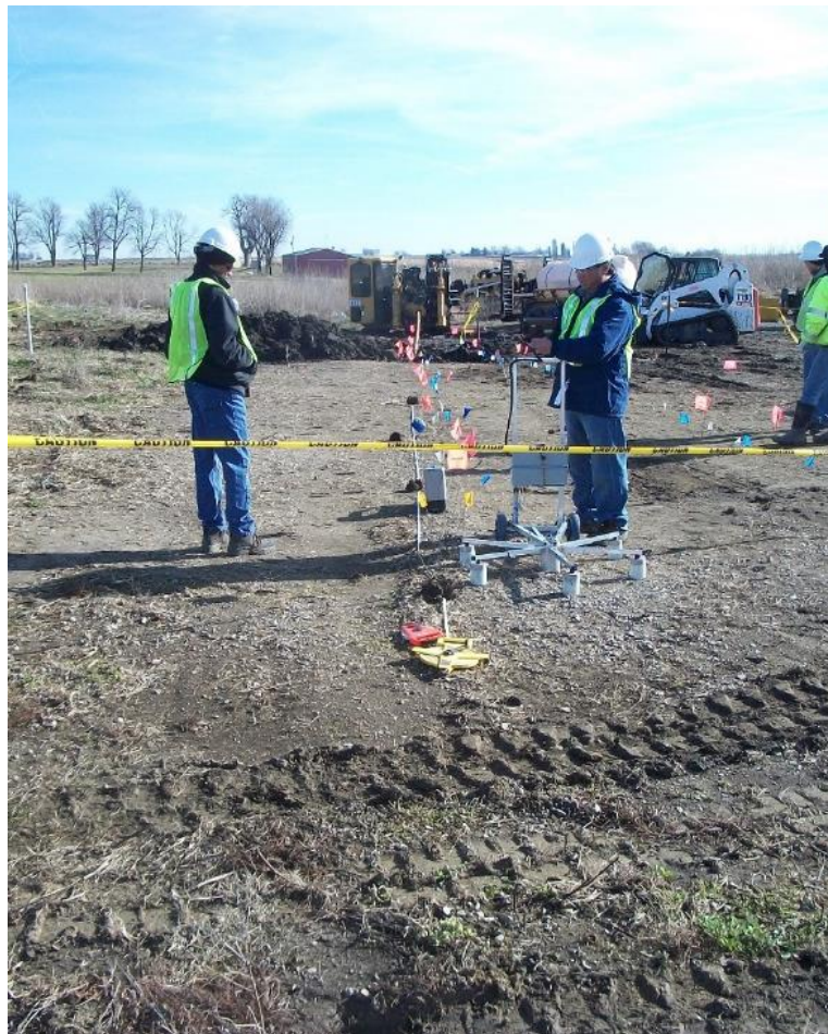
Figure 74 Photograph of the setup during December 2015 testing. Flags indicate the location of locator sonde positions, sensor, and source locations along the bore.
