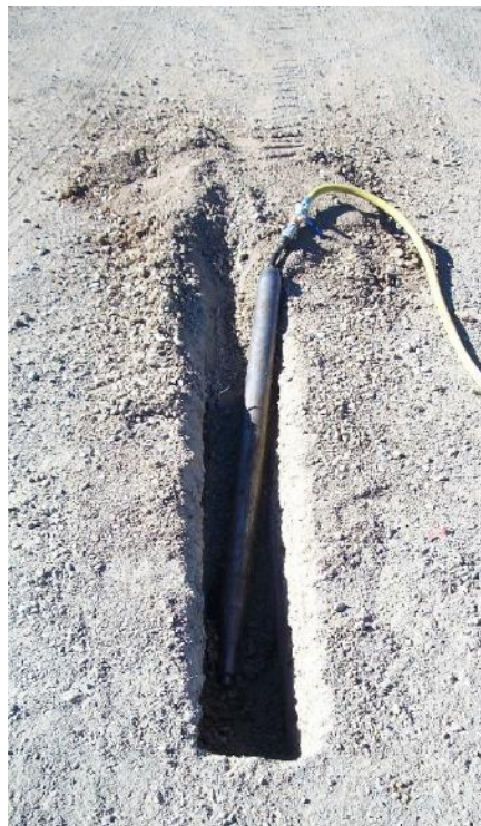
Figure 16 Photograph of a utility installation pneumatic 'mole'.
