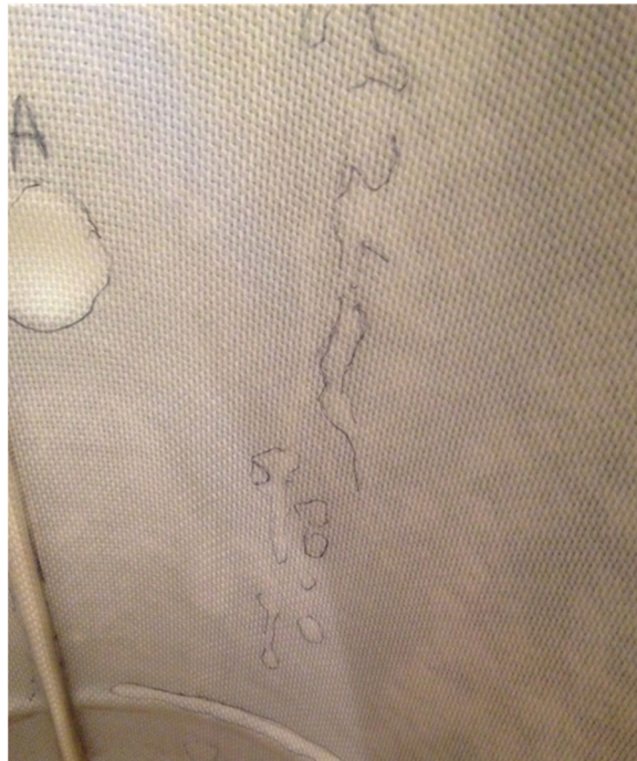
Figure 48 - Discoloration of the liner showing areas of possible voids before the test
