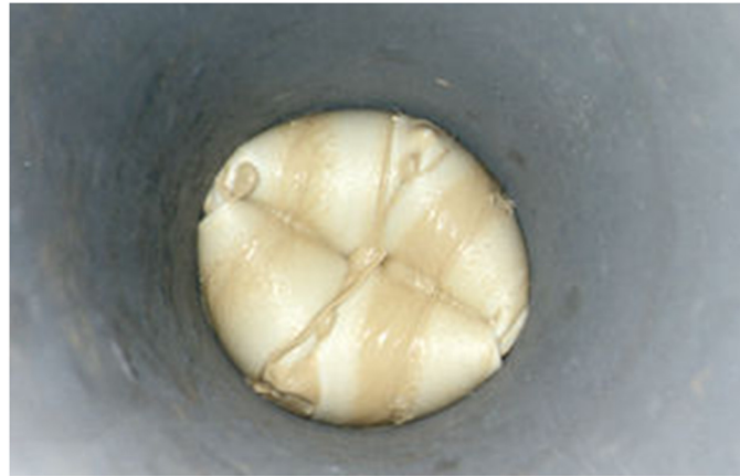
Figure 11 - Inverted-liner in the host pipe
