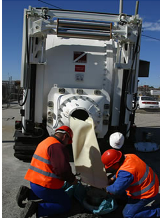
Figure 12 - Installation truck for the HPL-G Liner
