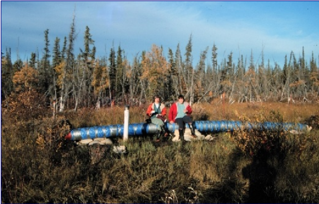
Figure B.2-1 – Upheaval of buried pipe, Norman Wells oil pipeline (Sept. 1997). The exposed pipe has since been covered by a berm ( http://gsc.nrcan.gc.ca/permafrost/pipeline_e.php )
