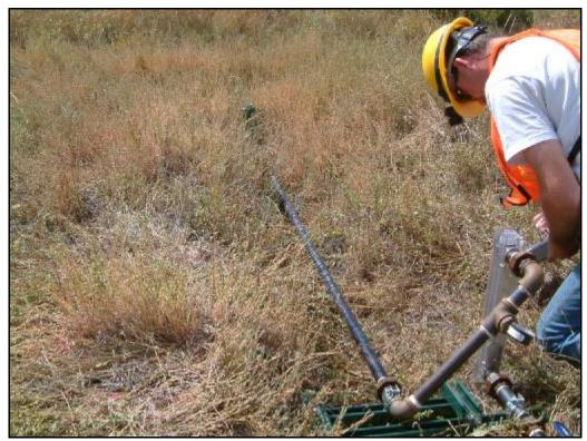
Site 3 – Aboveground leak at the end of the 10-foot long pipe.
